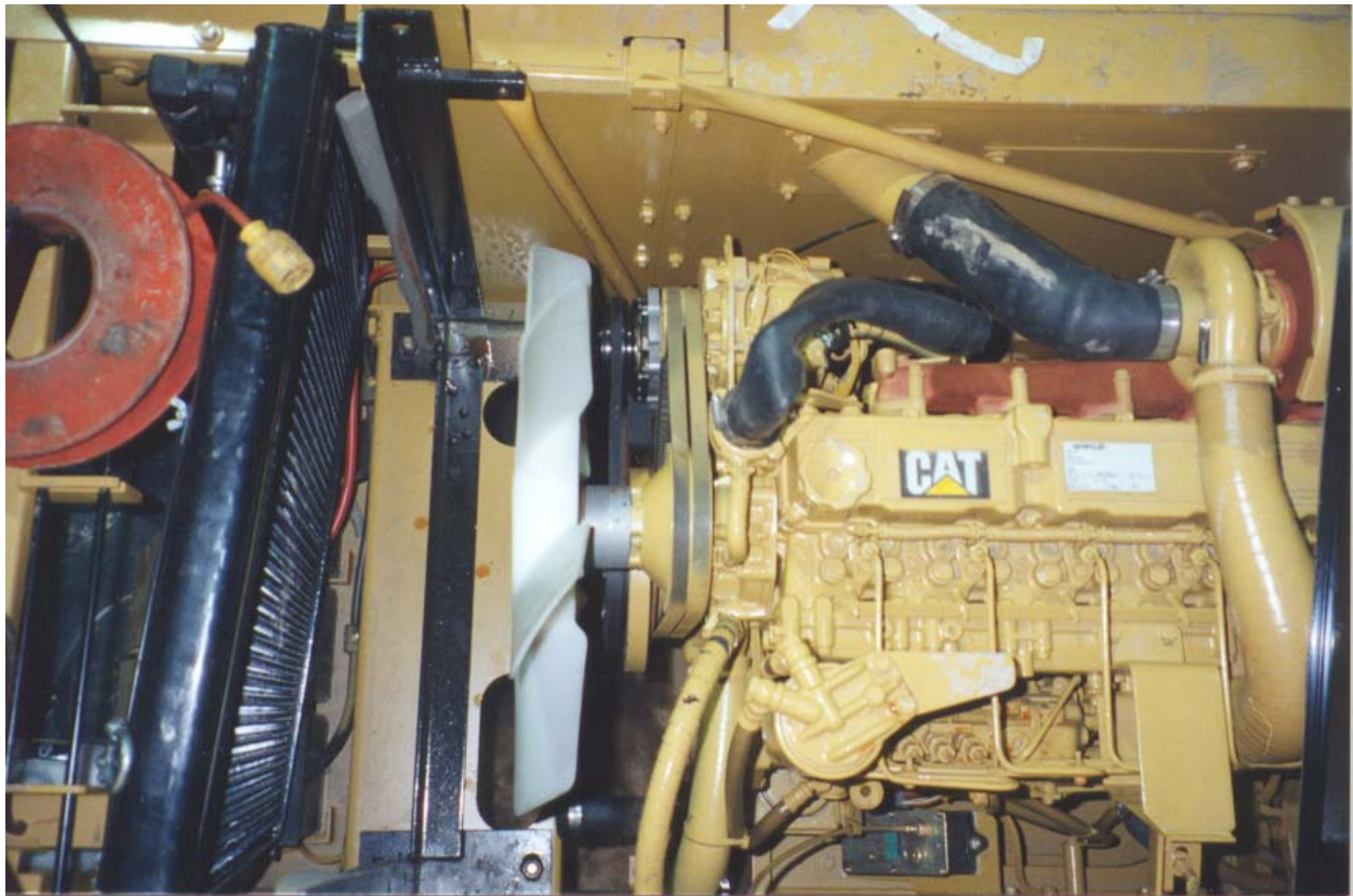
Compressor mount and drive in place on 315 Cat
